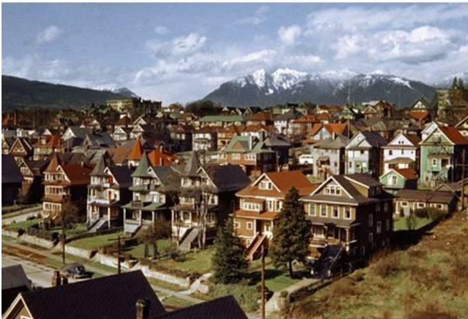
VIEW OF WEST END FROM BURRARD ST BRIDGE 1957
